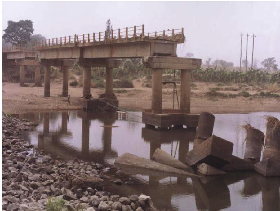
Fig. 2. A bridge damaged by floods in the Upper Niger River basin. Photo by: Andre Kamga Foamouhoue.
